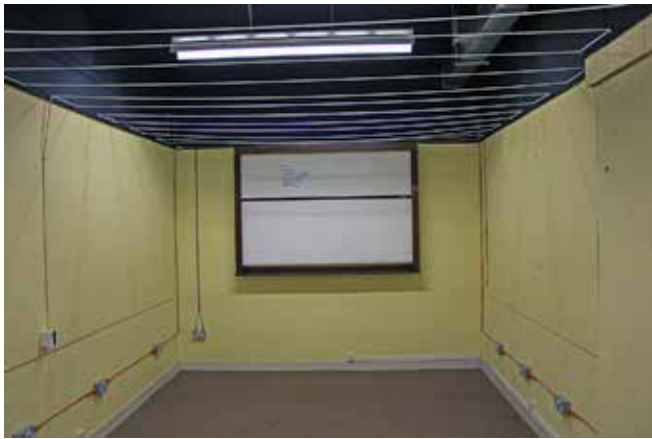
Council office, stripped of furnishings in 2018
